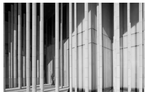
Figure 1. Image of the Pavilion
