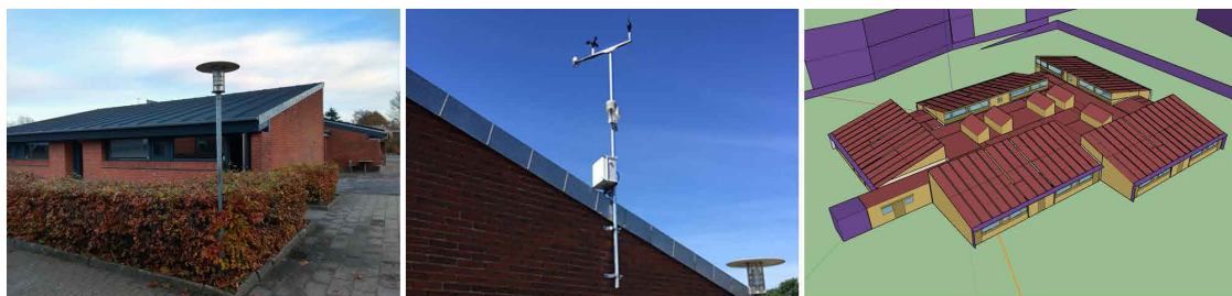
Figure 5. Library building from Gedved School, Denmark. Left: Outdoor image. Middle: Weather station installed on the building's roof. Right: The building energy model (OpenStudio plugin for SketchUp [64]).
